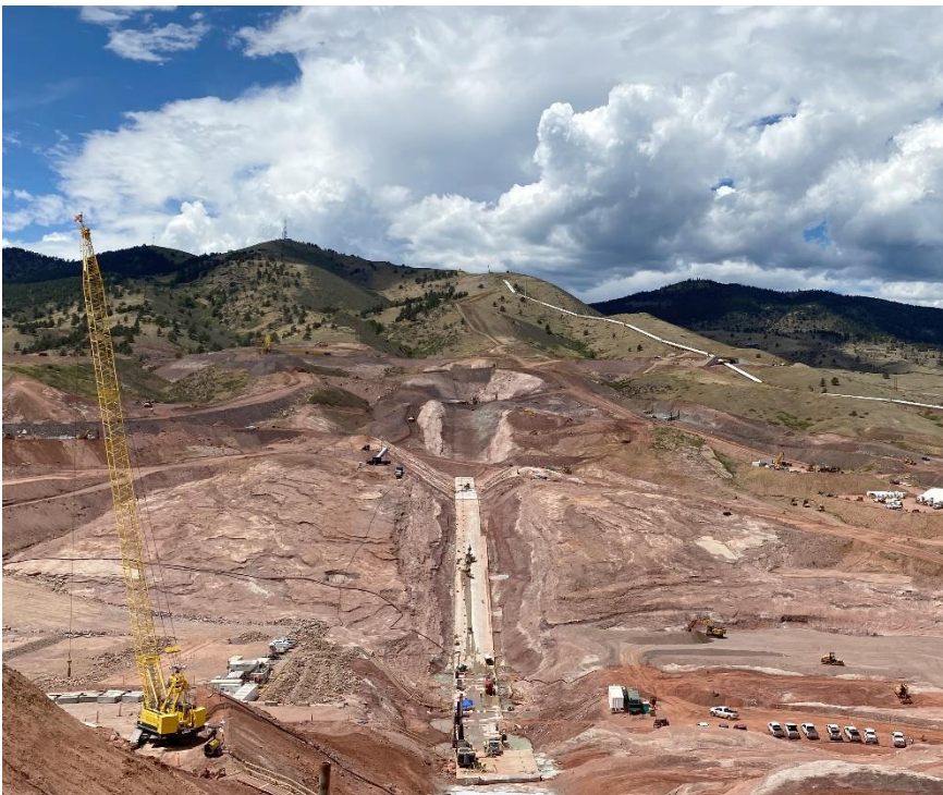
Construction progressed on the main dam at Chimney Hollow Reservoir in 2022.
